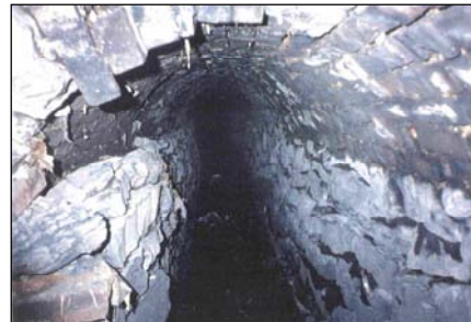
Typical Brick Arch Storm Drainage Tunnel
