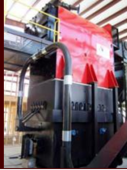
AFS Low Pressure Boiler (0-15 psig)
